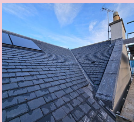
The High Street elevation just prior to works beginning. < left: Slatting has completed with leadwork and rainwater goods largely complete. Solar PVs are also installed, further adding to the sustainability of the new homes.
