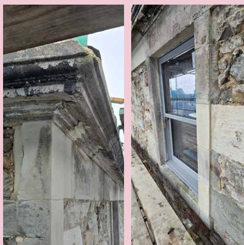
Stonework repairs are underway, utilising a range of specified techniques to restore the historic fabric BELOW: the Sparrow Terrace
