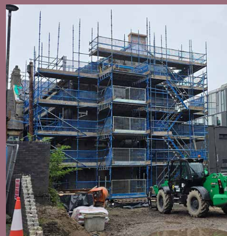
The rear elevation is taking shape with the roofs sheeted, the blockwork almost complete and the chimneys being installed. BELOW: Natural slate on-site and ready for installation in the next few weeks.
