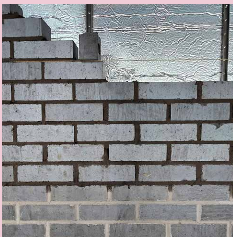
Nearing completion, brick and blockwork are completed in "lifts" of a number of rows per day, to avoid excessive compression of fresh mortar - hence the colour difference visible here. BELOW: Internal fit-out moving along.
