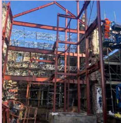
Steel frame nearing completion with temporary trusses showing/amongst
