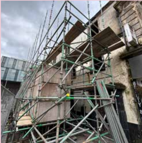
Temporary supports securing the historic façade
